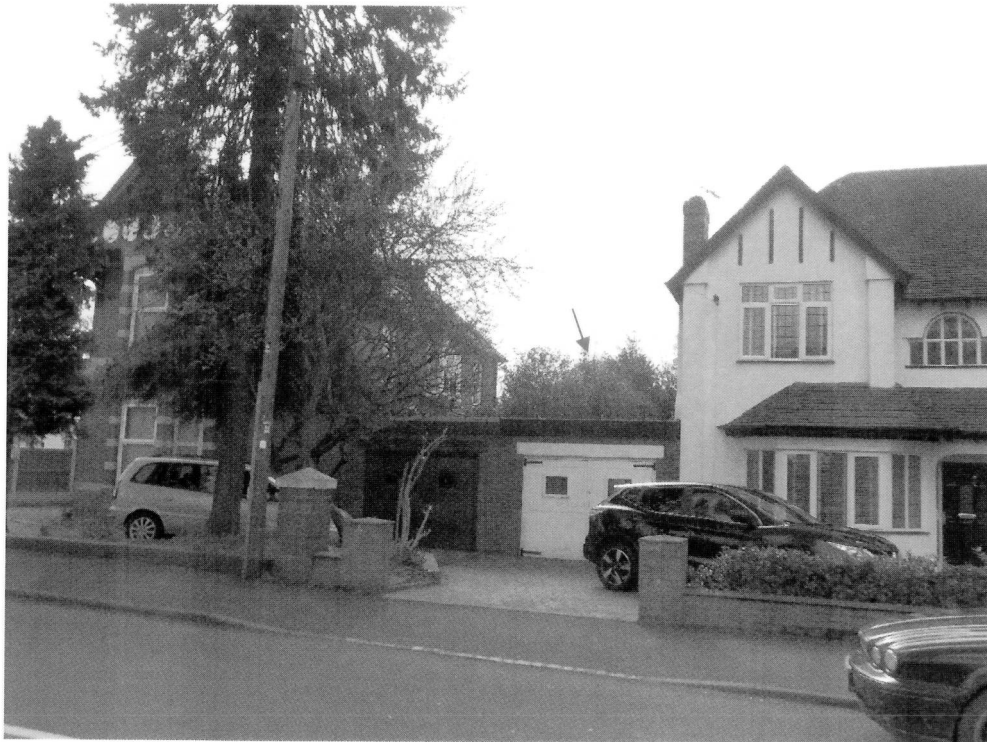
View from Station Road to front.
